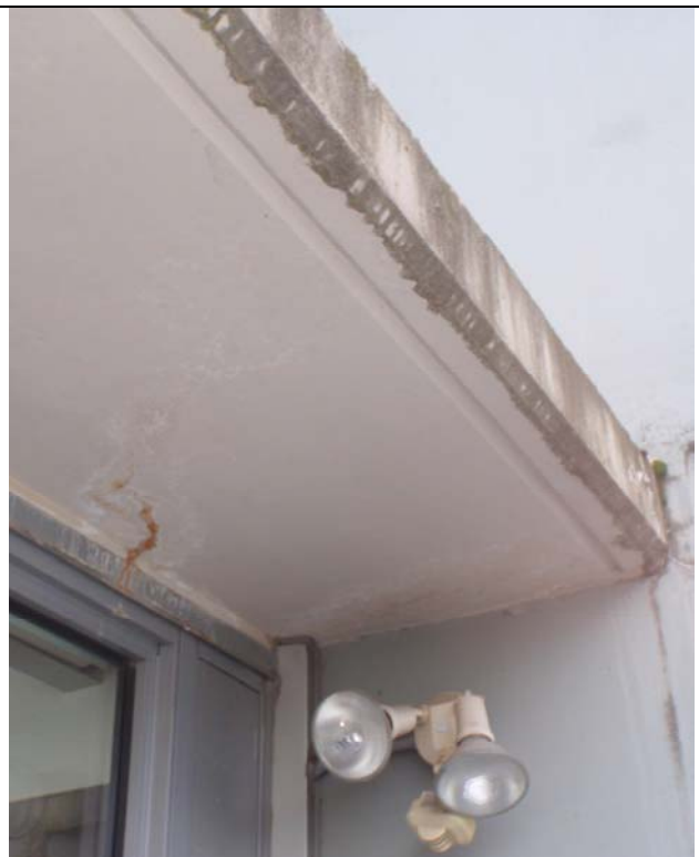
Photo # 20 – Cracking at unit 2801
