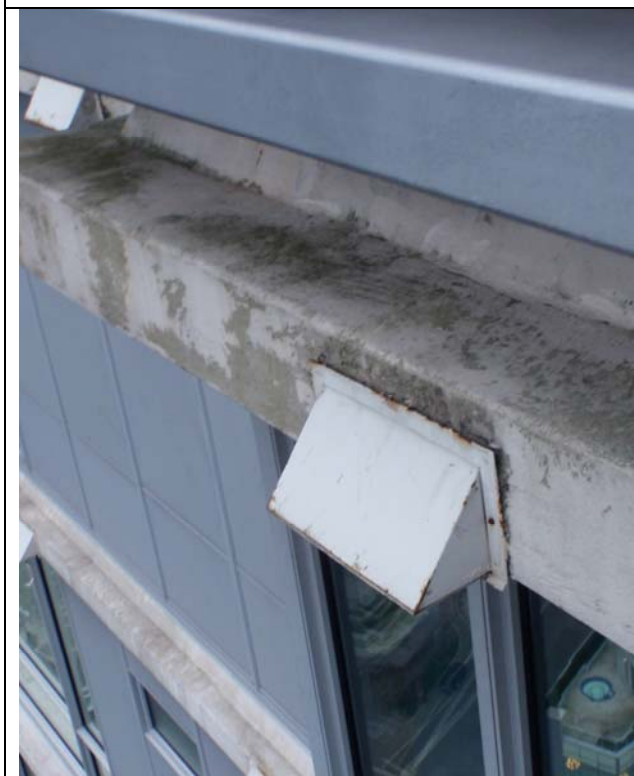
Photo # 11 – Paint peeling and missing sealant at vent cover
