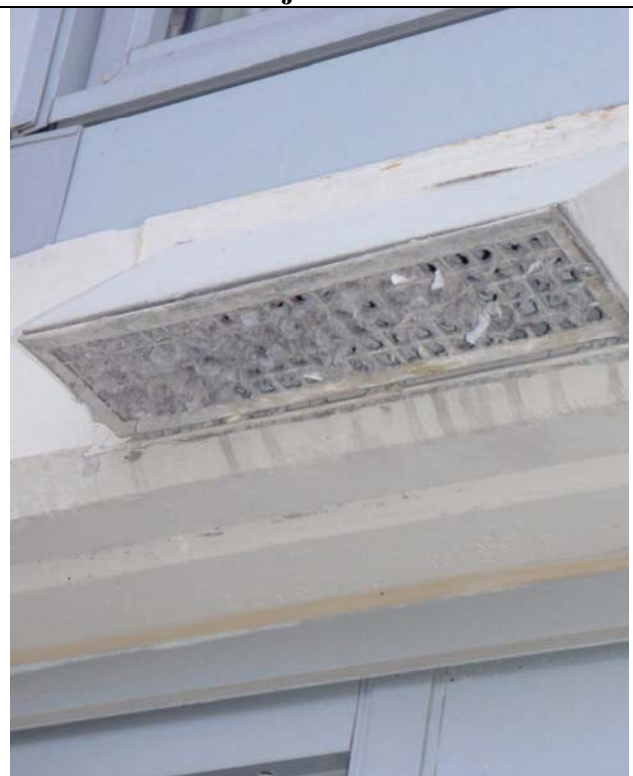
Photo # 16 – Plugged vent screen
