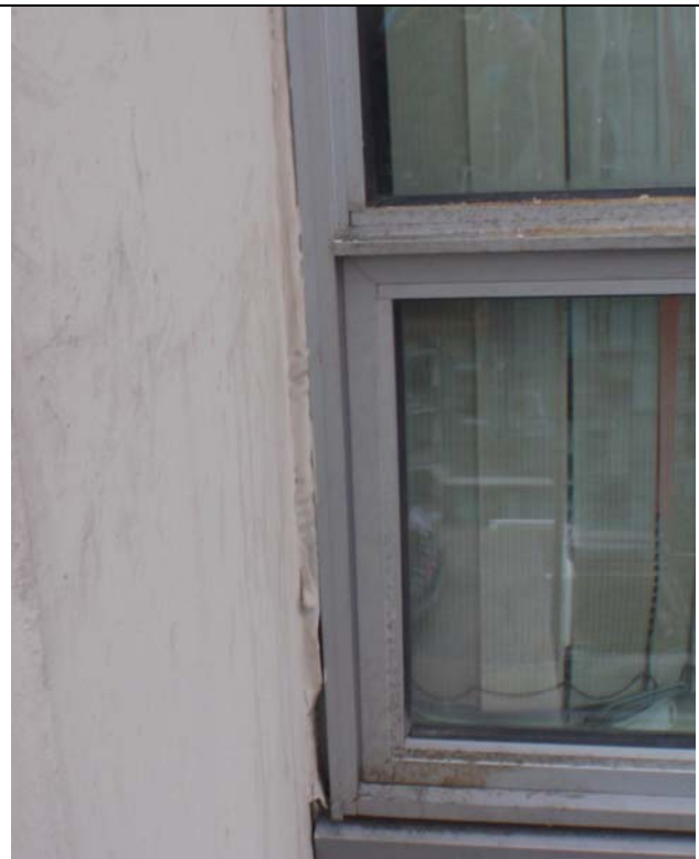
Photo # 14 – Sealant separation at window jamb
