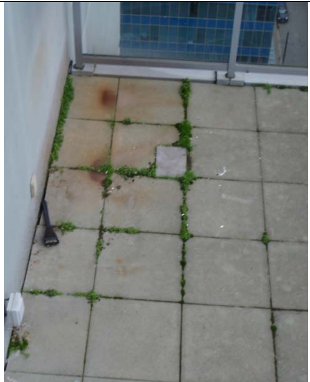
Photo # 2 – Organic growth on roof deck
