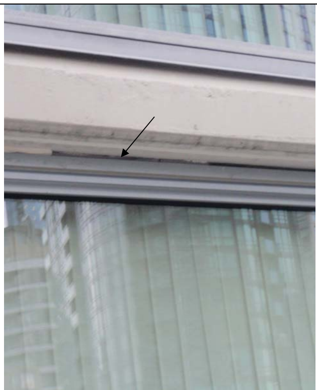
Photo # 12 – Missing sealant at window head
