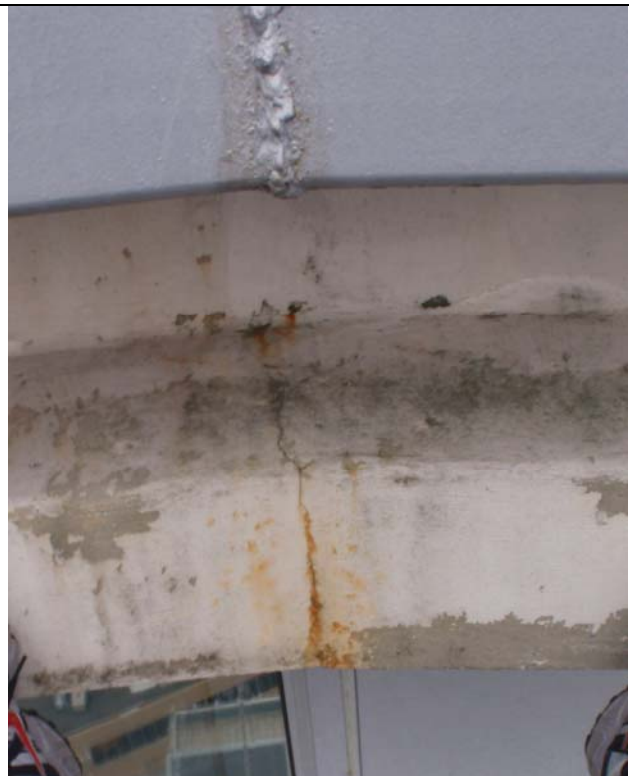
Photo # 8 – Crack in concrete
