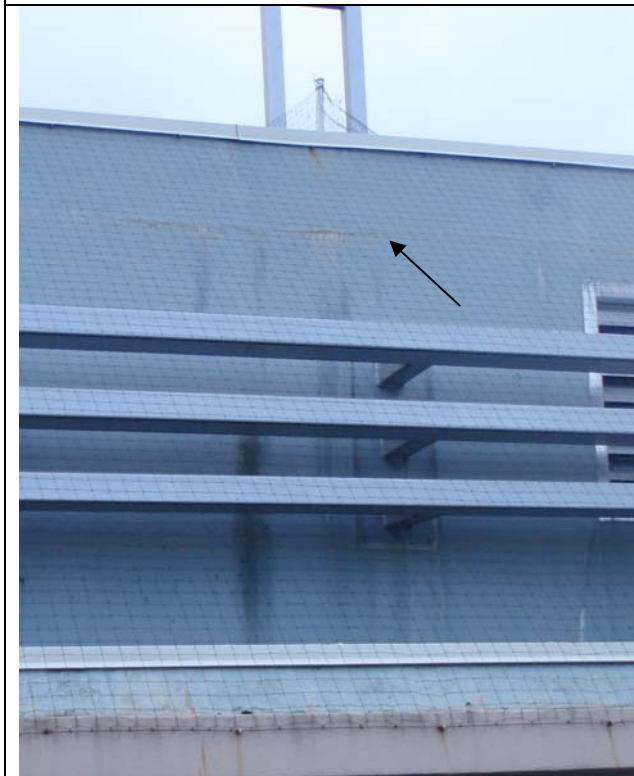
Photo # 7 – Horizontal crack in concrete
