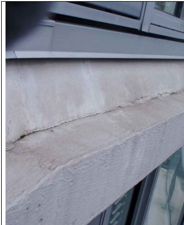
Photo # 9 – Horizontal crack in concrete
