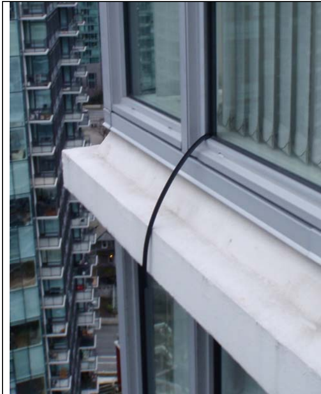
Photo # 5 – Loose window gasket
