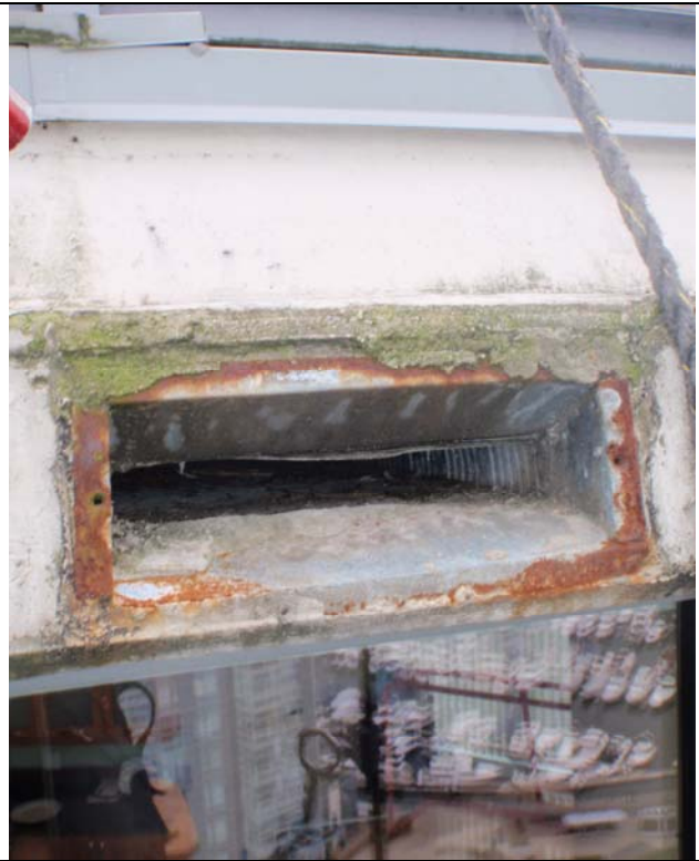
Photo # 18 – Missing vent cover
