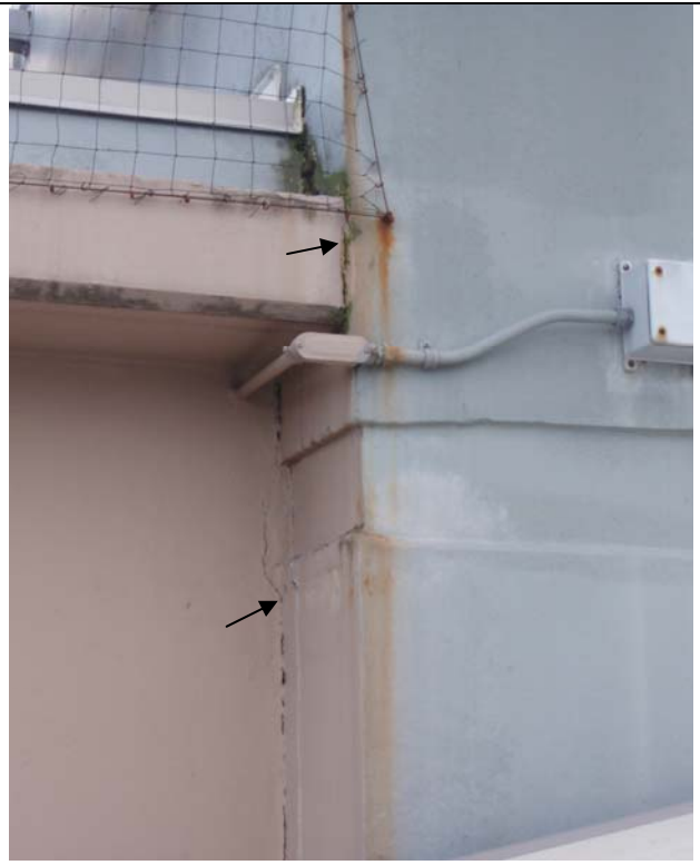
Photo # 6 – Cracks in concrete
