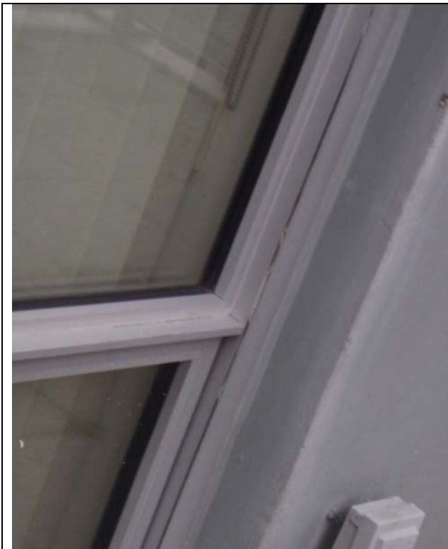
Photo # 13 – Missing Sealant
