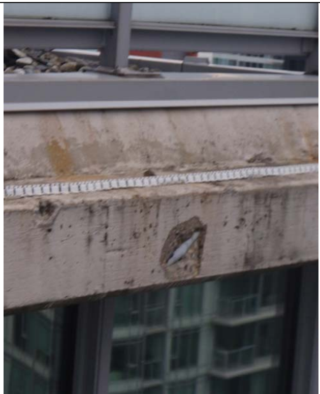
Photo # 10 – Chipped concrete
