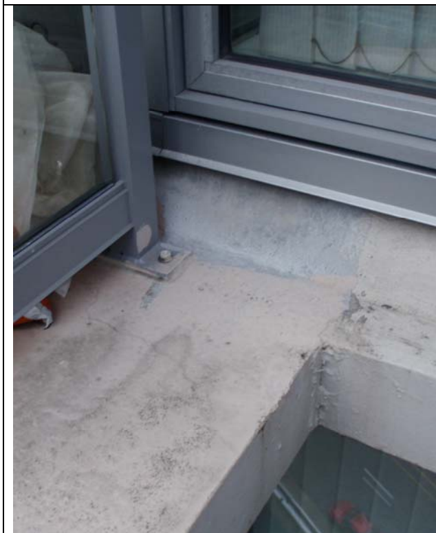
Photo # 3 – Missing membrane
